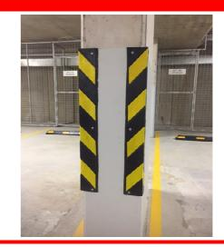
**FIXINGS** 6.5mm x 25mm Long - Counter Sunk Nylon Tap Ins (6 per corner guard)
